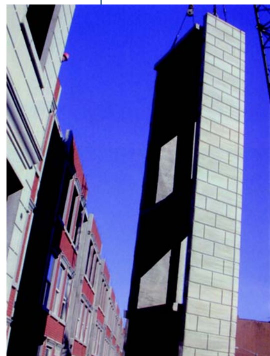
Precast Concrete homes built in the Bronx, NY
