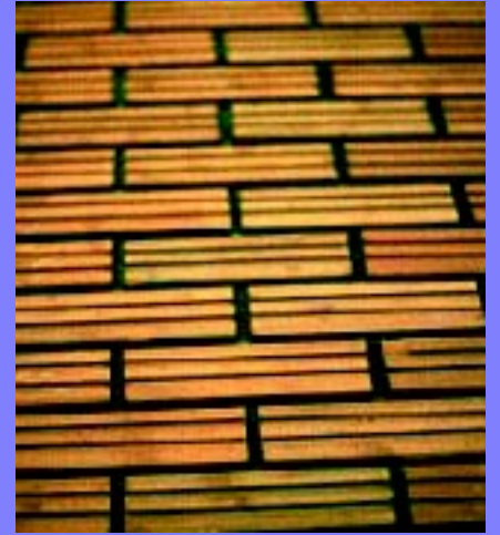
Thin brick installed face down in a gasketed formliner in precast mold
